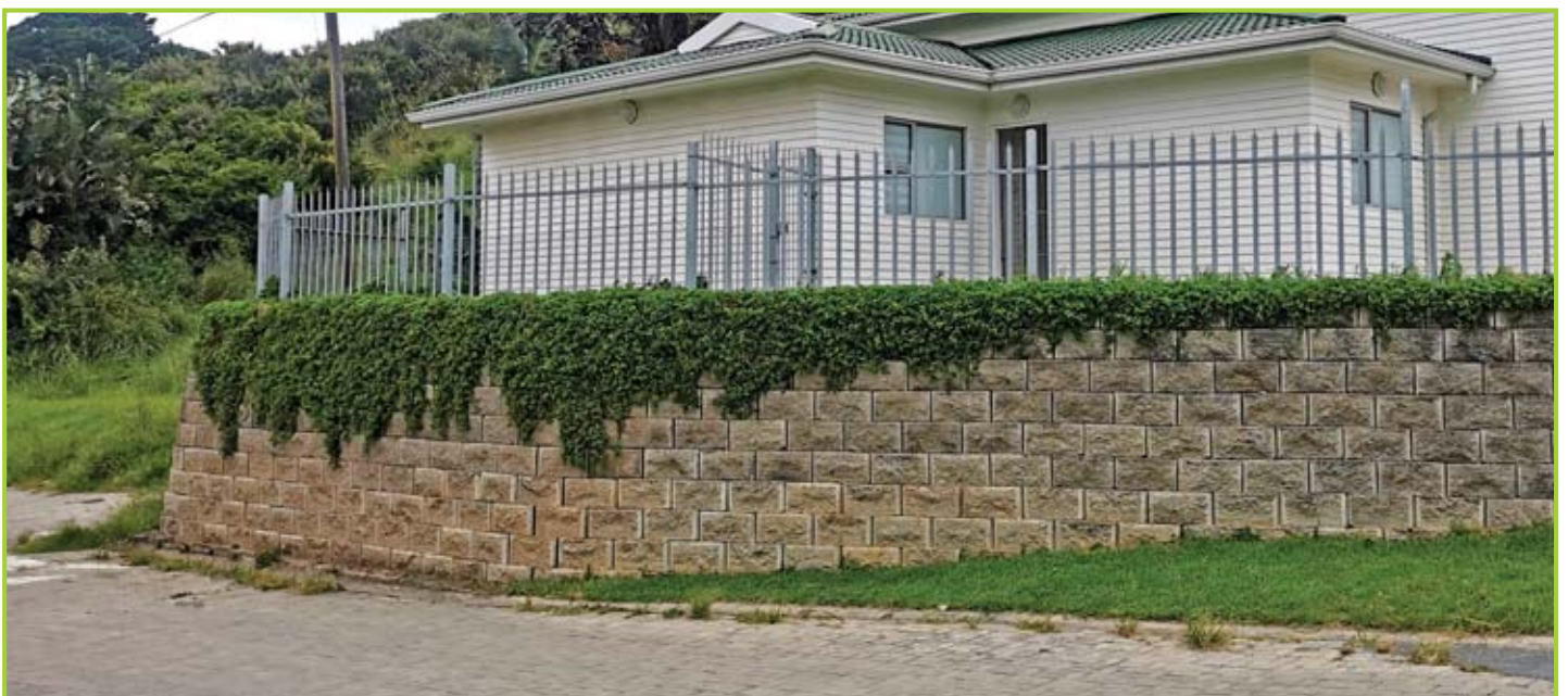
RECENTLY INSTALLED V10 ROCK FACE FINISH WALL
