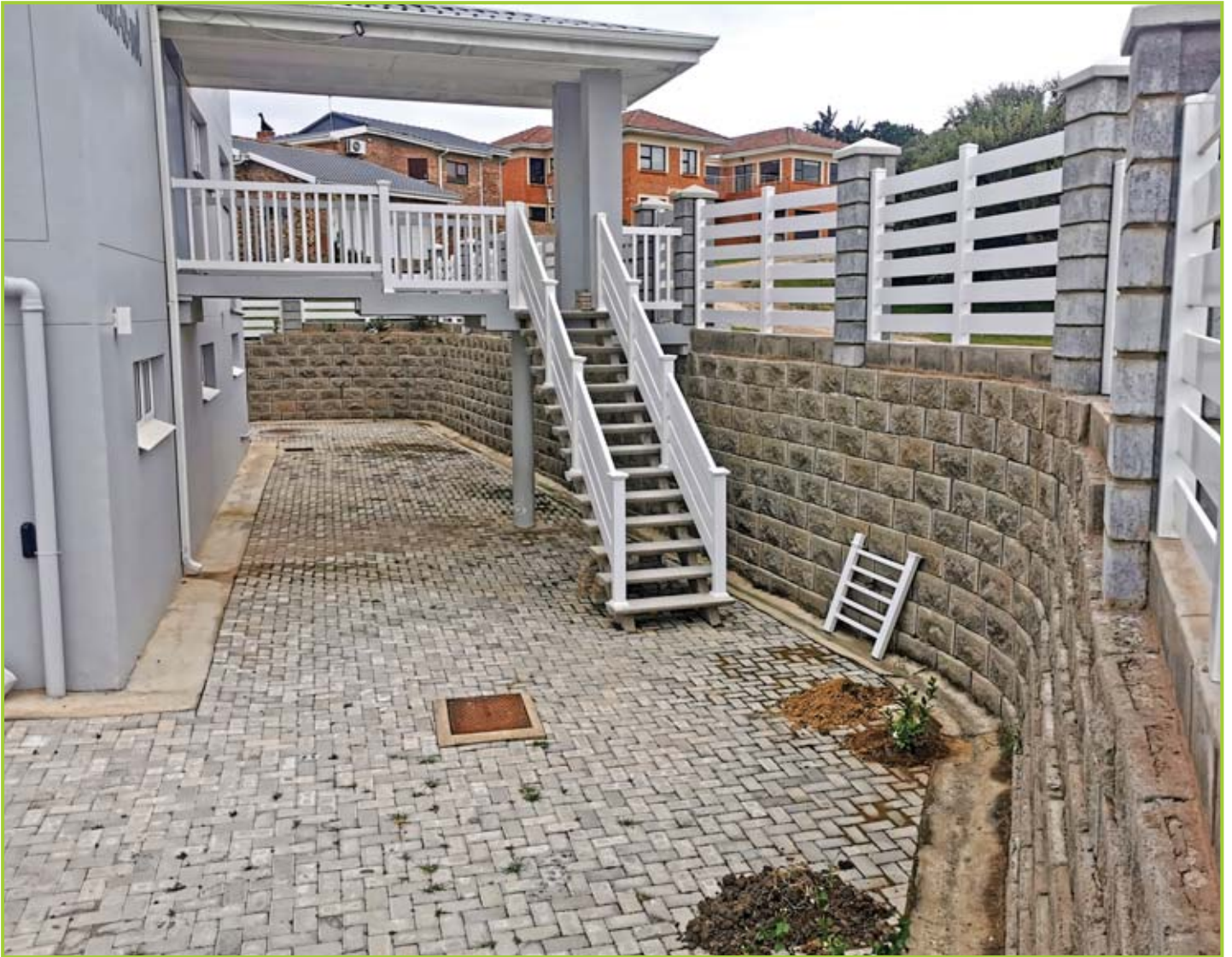
RECENTLY INSTALLED V10 ROCK FACE FINISH WALL
