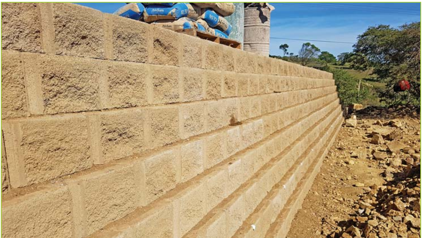
V10 BLOCK COMPOSITE RETAINING WALL (EARTH REINFORCED WITH GEOGRID)
